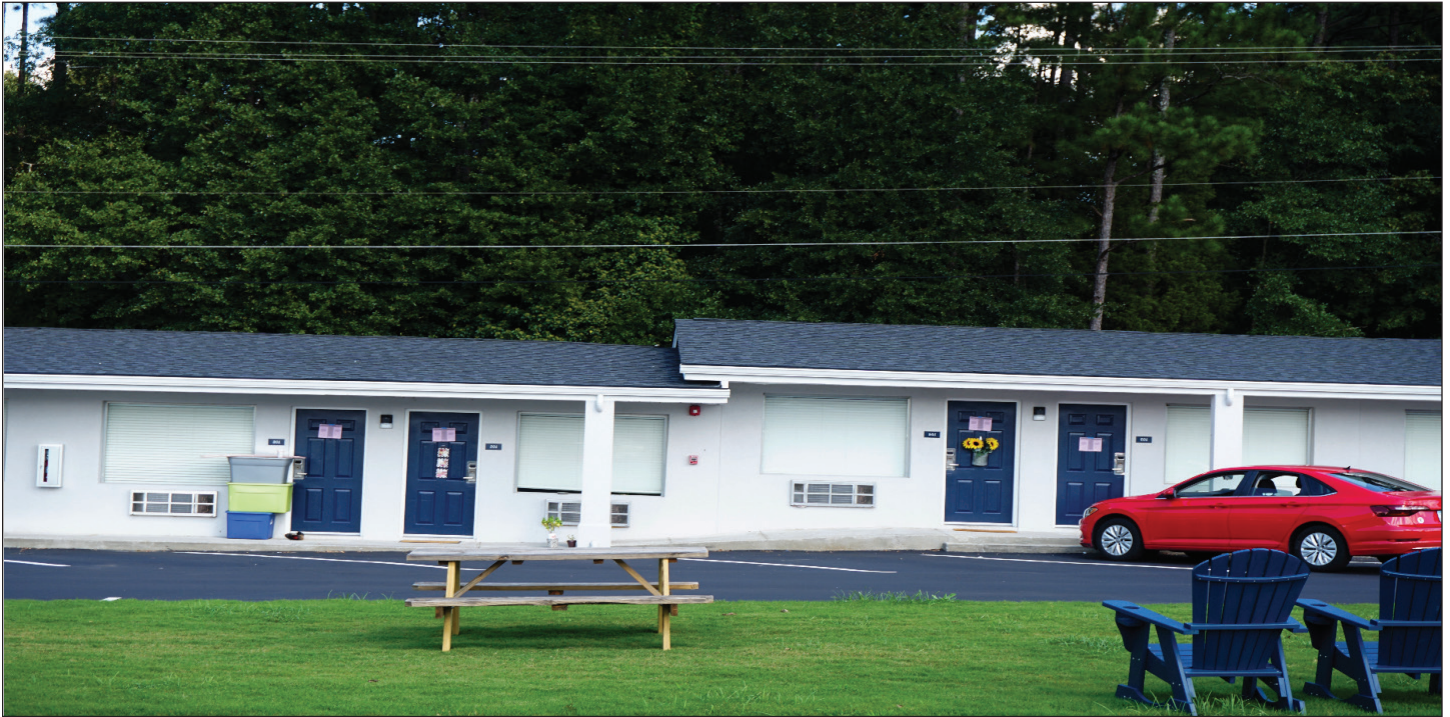
The newly renovated Oak Hill Residences.
